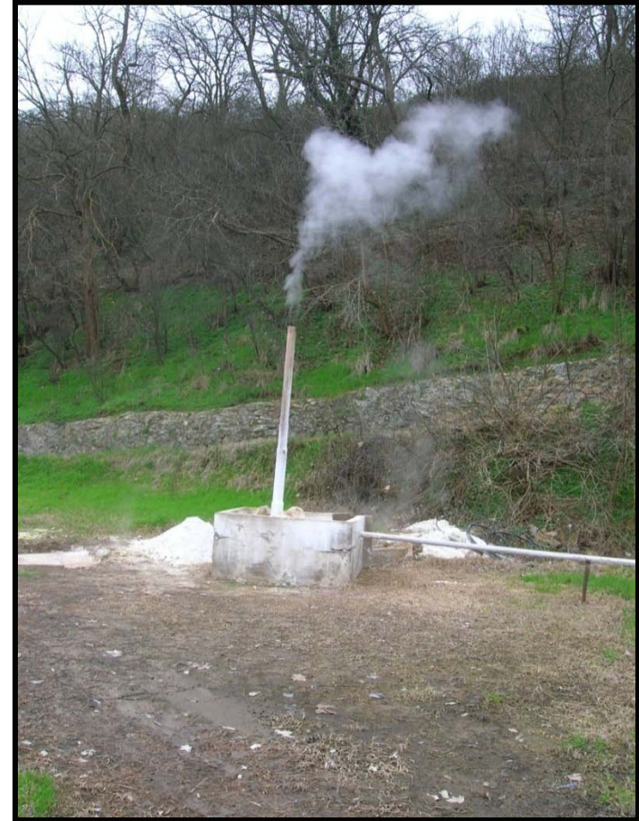
Existing Geothermal Well in the Vranjska Banja area
